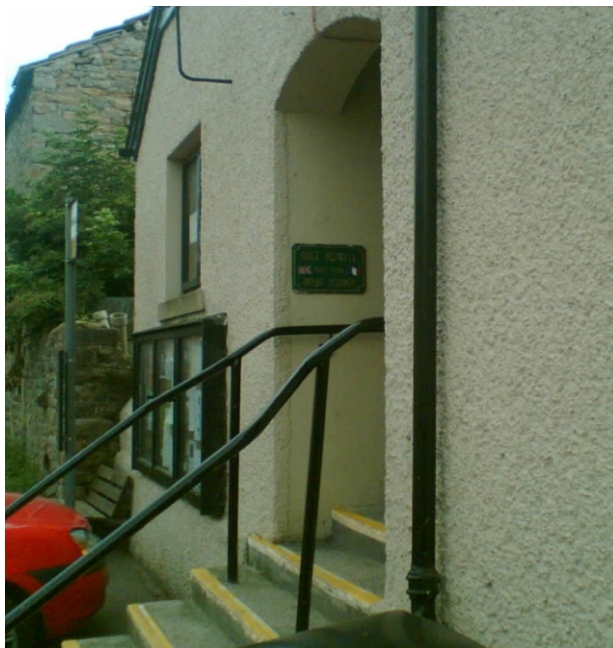
Fig. 2. Wray Village Hall, the site of the first display deployment.
